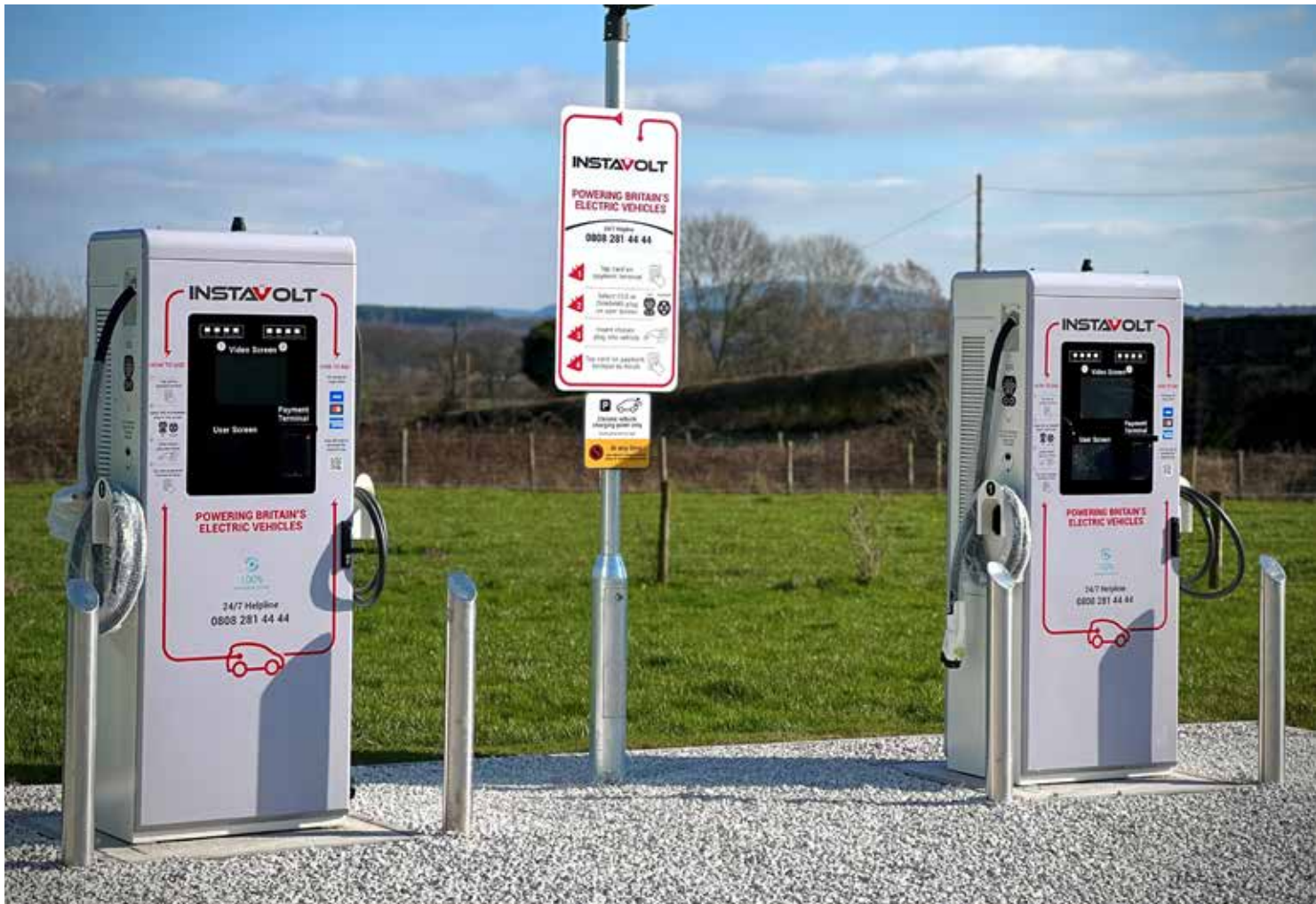
Two rapid 120kW chargers have been installed, which are capable of adding 100 miles of range to your electric vehicle in just 15 minutes
